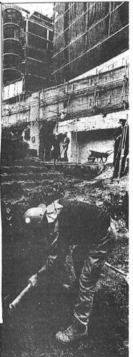
Digging in... at Spitalfields cemetery in Bishopsgate
