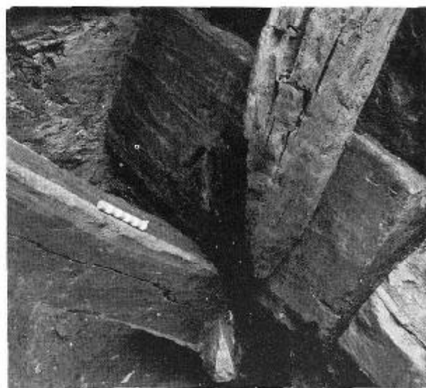
Fig. 6. Details of carpenter's mark on back of sill-beam.
