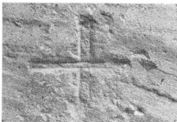
Fig. 6: Mason's mark and tool marks on the interior face of the outer wall of the Wren Church of Christ Church.
