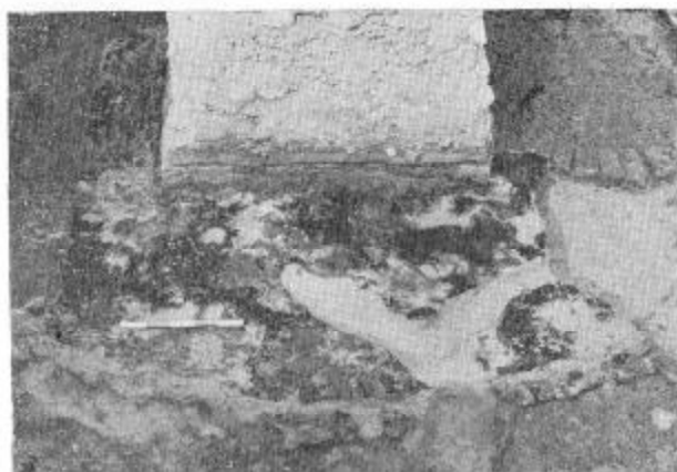
Fig. 4: Scorched destruction of building D, looking west.
