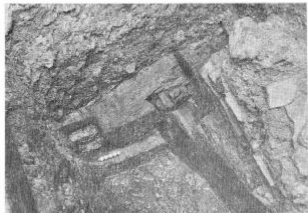
Fig. 7: Tieback of 1st century Roman quay projecting south of quay wall to the east of the timber-lined drain.
