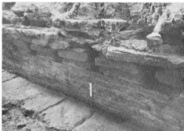
Fig. 5: Brick-lined culvert under floor of Building A.
