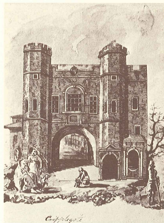
Medieval gate at Cripple Gate, in the 18th century. In this form it probably dates from a rebuilding of 1491 when Edmund Shaa, goldsmith and mayor, bequeathed 400 marks for its repair. Its design, with octagonal towers, low arch and string courses running along the façade, is similar to the south gate at King's Lynn, designed by Richard Hertanger of London in 1437.
