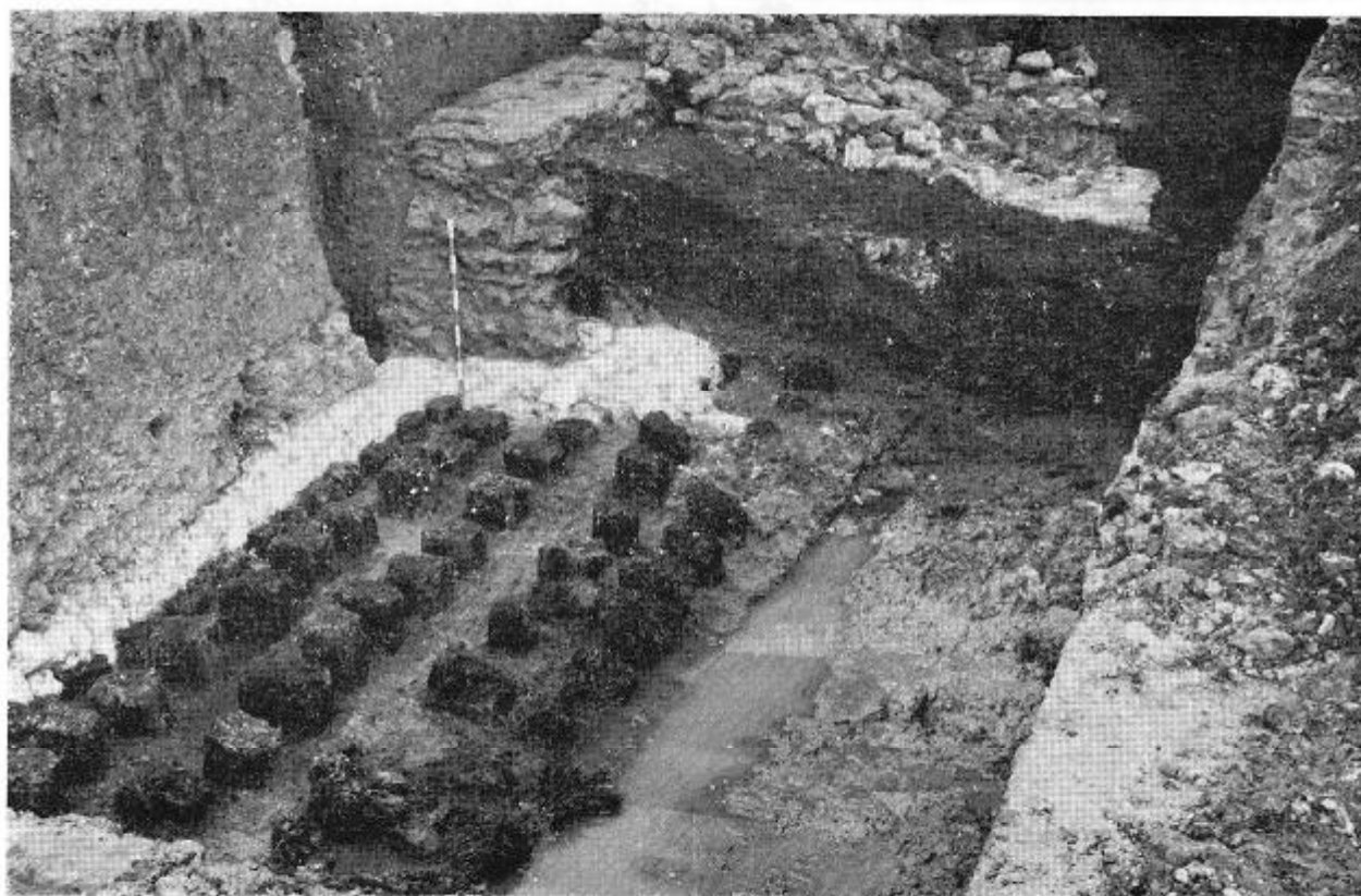
Fig. 1. The foundations of the wall showing the oak piles cleared of their chalk packing; two of the tile courses are also visible. (Photo: Trevor Hughes, Guildhall Museum, D.U.A.)
