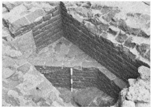
Fig. 5: The foundations of a polygonal stair turret with its Reigate stone dressing. The palace wall is top right and the 17th century rebuild which "housed-in" the stair turret is bottom left.
