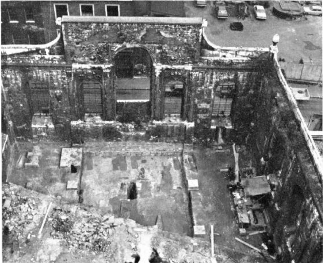
Greyfriars; view from west showing area of excavation and east end of the Wren church
