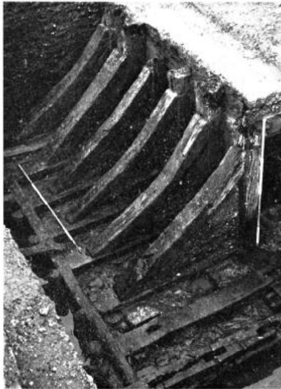
Plate 6.—Custom House site; Trench IV, later Medieval quay from the south-east (scale in 0.5 m.)
