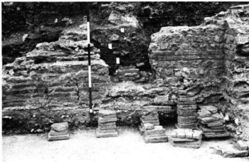
Plate 6. Huggin Hill baths: North-east corner of Room 30 viewed from the south showing the 'mock ashlar' wall to the right of the flue containing a pila opening into Room 32. Scale of feet.
