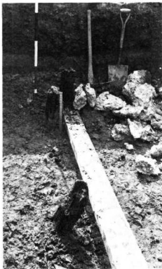
Plate 1. Queen Street, 1953 & 1960: Timber piles, Feature 21.
