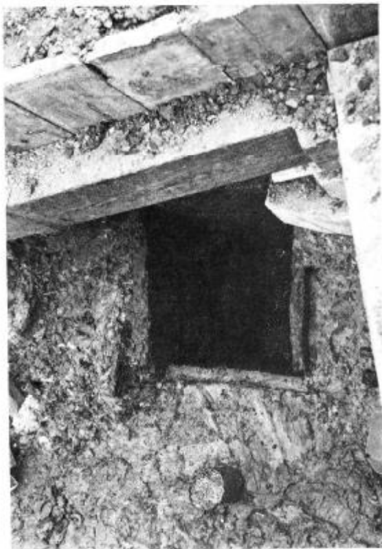
Plate 3. Queen Street, 1953 & 1960: Upper timbering of Well 20.
