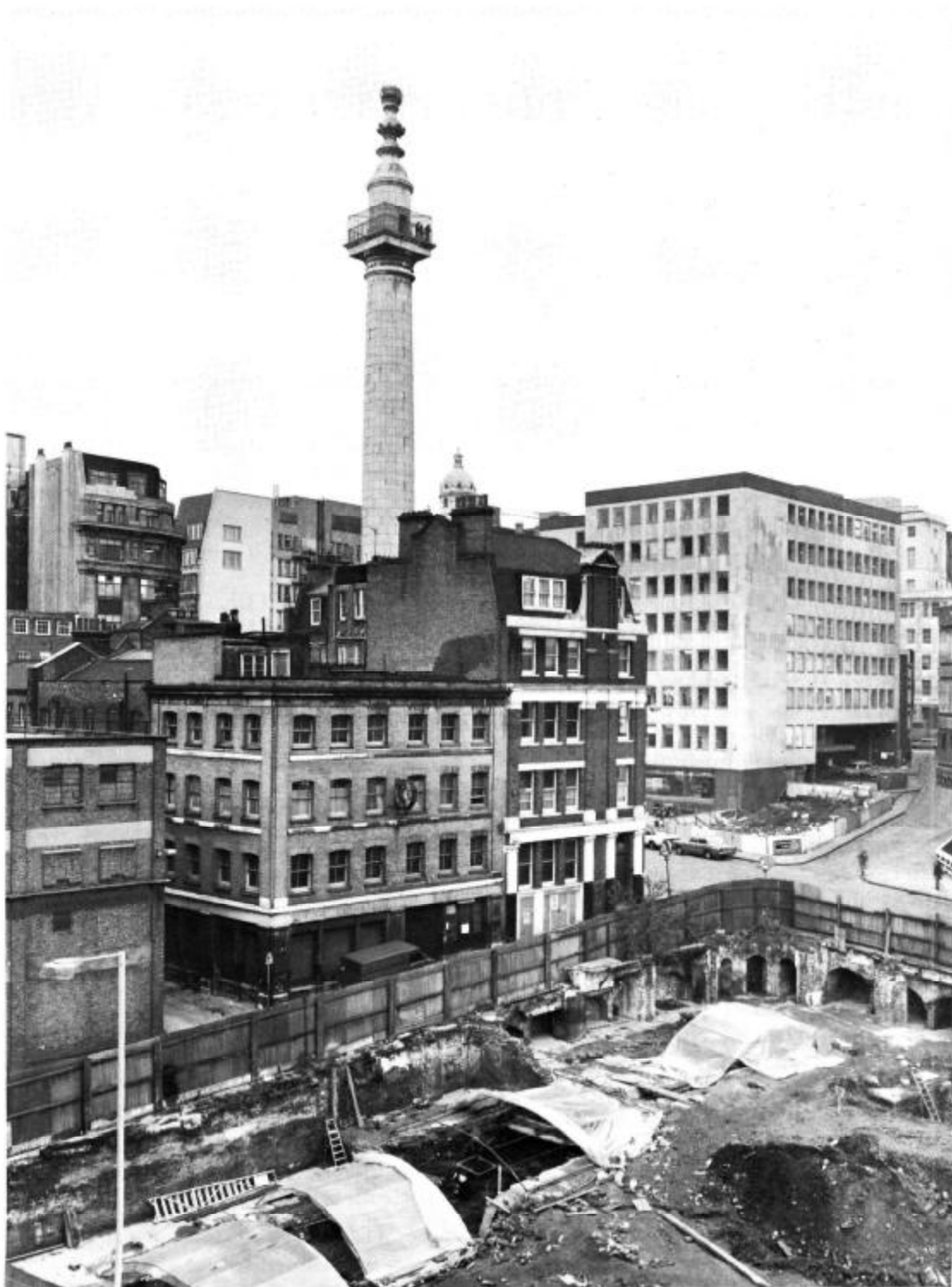
Fig. 1 Pudding Lane: Excavating on the Peninsular House site, Pudding Lane, in the shadow of the Monument. The polythene cover on Area B has been rolled back revealing the cellar of a building burnt in the Great Fire of London.
