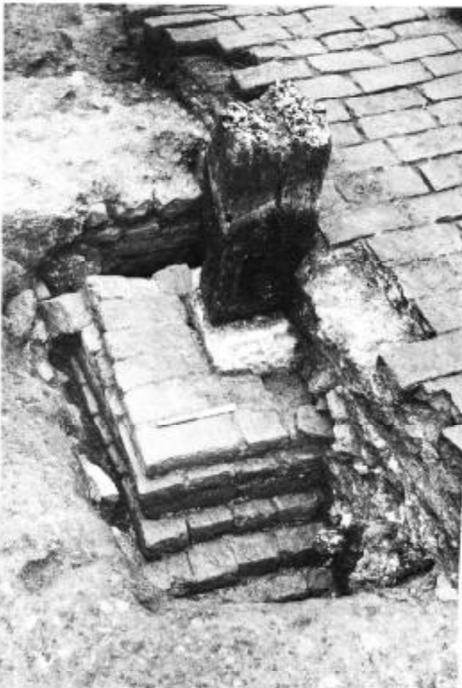
Fig. 5 Pudding Lane: Detail of sub-surface brick plinth on which posts supporting the ground floor were set: 2 × 100mm scale.
