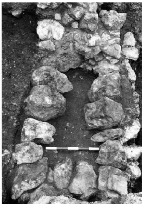
Fig 55. Milk Street: Building 6, details of the construction of the south wall, looking west. (a) large boulders of ragstone were laid to form the outer skins of the wall, on the chalk foundation; (b) the core was infilled with chalk, flint, and fragments of Roman tile, all mortared. Scale is 5 × 100mm.
