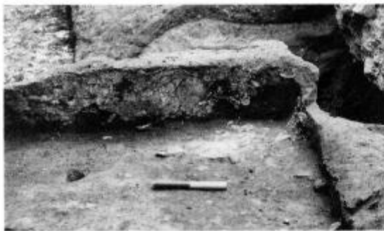
Fig 34. Building 6, Leadenhall Court site (LCT84): traces of plaster rendering on internal face of brick wall
